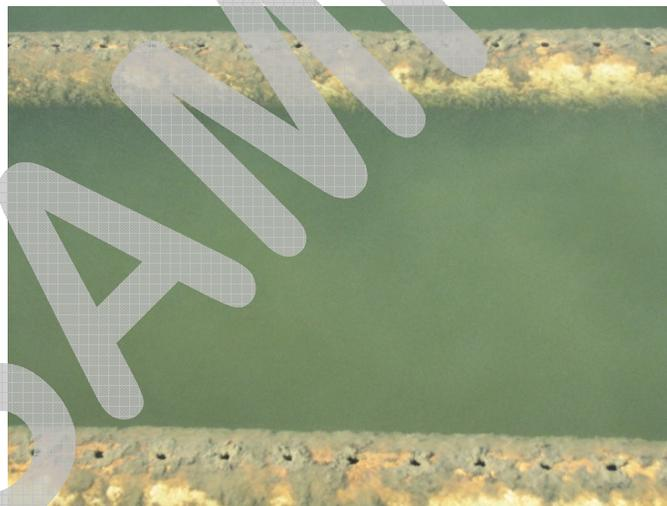
**Figure 2-4 – Pin Floc in Settling Basin of SuperPulsator**
